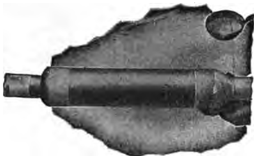
FIG. 7.405.—Cable splicing with Oxite: 6. Placing lead sleeve in position and wiping the joint. Move lead sleeve into proper position so that each end equally overlaps the lead sheathing of the abutting cables. Press down ends of sleeve to fit snugly around cable sheathing. Wipe joint between sleeve and sheath carefully with edges of wipe at least \frac{3}{4} inch from the line at which the sleeve and sheath meet. Cut two holes, one at each end and on top of the lead sleeve. One of these is for pouring in the hot compound and the other for its overflow. The one selected for filling should be on the end farthest away from the paper tubes and so located that the stream of hot compound will strike the belt insulation of the jointed cable.
