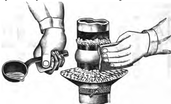
FIG. 8,606.—Method of wiping a vertical joint. A small piece of cardboard cut open is placed under the joint to catch excess solder, or as shown, a lead flange cut open is placed around the pipe and held in place by twine.
