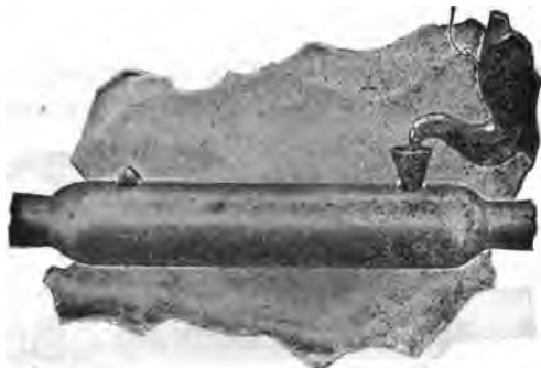
FIG. 7406.—Cable splicing with Ozite: 7. Filling and completing the joint. Before pouring in the hot "Ozite", the joint should be slightly tilted so that one end will be slightly higher than the other. As it is necessary to pour the hot insulating compound into the hole at the lower end of the joint, an iron filling cup, one end of which is belled out to make a funnel, should be screwed into the filling hole at the lower end of the joint. This cup or funnel must be long enough to bring its top on a higher level than the overflow hole in the other end of the sleeve when the joint is in the inclined position. The object in placing the joint in this inclined position and pouring the compound into the lower end is to drive all air and moisture upwards in the natural direction and away from the soldered joints, the hand applied insulating tape and tubes. The "Ozite" insulating compound having been heated to the pouring temperature indicated on the label on the container (which temperature should be determined by thermometer) it should be poured slowly and steadily into the filling funnel at the lower end of the lead sleeve. At least two or three gallons of compound should be allowed to flow through the overflow hole or until the portion overflowing is entirely free from bubbles. The joint should not be allowed to settle for at least four or five hours cold, covered with a canvas pad, oil cloth or other protection from cold air, dirt moisture, etc., and to prevent chilling too rapidly. When the joint has cooled sufficiently to prevent cracking of the soldered wipe, the lower end should be raised so that the joint is level, for further settling, and the joint placed in its permanent racked position. The joint having thoroughly settled and cooled, refill it through the same filling hole as before so as to fill up all air spaces due to shrinkage in the original filling. Solder up the filling holes and the joint is completed.
