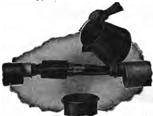
FIG. 7.402.—Cable splicing with Ozite: 4. Boiling out tape and cable ends. Fill space between ends of copper connector and conductor insulation on each side with loosely woven and easily impregnated cotton tape. Apply similar tape in one layer over the copper connector for its entire length. Boil out tape and adjacent cable ends carefully with "Ozite" insulating compound. As the tape must have its moisture boiled out, in case any be present and be thoroughly impregnated besides, nothing but very hot compound will suffice.
