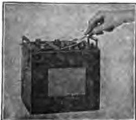
FIG. 6,341.— Battery repairs 41. After the form is removed there is always an excess of sealing compound. This can be scraped off with a hot putty knife.
