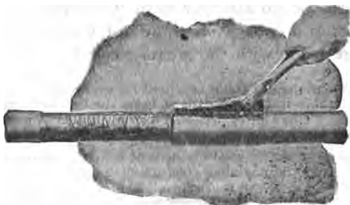
FIG. 7.399.— Cable splicing with Ozite: 1. Removing the lead sheath. The cable ends having been brought into position and cut off square so as to just nicely butt together, they should be marked at the point to which the lead is to be removed which should be approximately 7 inches back from the end of one cable and 10 inches back from the end of the other. At the points marked, the lead should be scored or cut entirely around. (Experienced jointers accomplish this result with a plumbers chipping knife and hammer.) The lead is then cut lengthwise of the cable, from the circular score to the end with the chipping knife and the piece of lead removed with a pair of pliers. Caution: great care must be exercised in removing the lead so as not to injure the cable insulation. The circumferential cut should be made by nicking the lead only part way through and then tearing or pulling it apart with pliers. The longitudinal cut should be made by inserting the knife tangentially with the inside curve of the lead sheathing, that is, so that the knife will pass between the insulation and the lead and not cut the insulation. After the lead has been removed, the edge of the lead sheath where it was scored should be carefully examined and all sharp edges or projections which might penetrate the cable insulation, removed with a knife. The ends of the sheath should then be slightly belled out, using some blunt instrument such as the end of the pliers..
