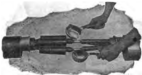
FIG. 7,401.—Cable splicing with Oxite: 3. Putting on lead sleeve and paper tubes, and sweating connectors to conductors. The lead sleeve which will later be used for jointing should be thoroughly scraped with a shave hook or rasp for about 2 inches and the cleaned portion thoroughly smeared with some convenient flux (usually stearine) which, by preventing formation of the usual film of lead salts, insures a close union between the lead and the wiping metal which is used to make the joint between sleeve and cable sheath. Thread the lead sleeve, prepared as described above, over one of the abutting ends of the cable and move back out of the way. Thread large enclosing joint tube, when used, over the cable end and push back out of the way. Thread small jointing tubes over the individual conductors of the longer cable end and push back far enough to leave the bare conductor ends easily accessible. Sweating connectors: Insert ends of conductors to be joined into the split copper connectors opened slightly, which should preferably be of such size that even when compressed upon the conductor the longitudinal split will remain open \frac{1}{16} or \frac{1}{32} of an inch. Pour hot solder from the ladle over the copper connector keeping the split in connector uppermost and, after thoroughly heating, compress the sleeve. Then sweat the connector and conductor thoroughly together keeping the joint as full of solder as possible. Wipe off all fins or points before solder sets. Do not file off fins or sharp points unless the copper connectors and the insulation of all of the conductors are protected from falling particles of metal. Do not move the copper connector or joint until thoroughly cooled, otherwise the solder, if it be at the critical temperature when mealiness appears, may not unite the parts satisfactorily.
