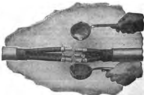
FIG. 7.400.— Cable splicing with Ozite: 2. Removing the insulation and tinning the conductors. Remove belt insulation of cable to a point about 1\frac{1}{2} inches from the edge of the lead sheath. The inner layers of belt insulation should be torn rather than cut so as to avoid damaging insulation of individual conductors. Pull jute fillers back and cut off at a point close to end of belt insulation. The individual conductors will now be found to be about 3 inches longer on one cable end than on the other. Strip the individual conductors of insulation for a distance equal to \frac{1}{2} of the length of the copper sleeve. Tin conductors thoroughly with hot solder applied with a ladle as shown.
