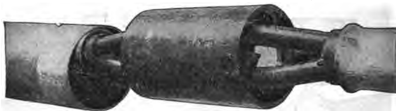
FIG. 7,415.—Cable splicing with Conducell: V. Joint insulation assembled and ready for the outer lead sleeve to be slipped over and wiped in the usual manner. Filling the joint: To insure a completely filled joint, experience has shown that unless facilities are provided for the escape of the gases, which are produced when pouring all compounds, an efficient and homogeneous filling cannot be assured. For this reason the openings through which the joint is filled should be large so as to permit of the compound being readily poured and also to provide means for the free escape of the gases. Further, it is desirable to provide means for raising the level of the compound above the level of the lead sleeve so as to insure that the joint will be completely filled. As a ready means for providing large filling holes and a higher level for the compound the special tools shown in figs. 7,417 to 7,420 have been devised. In filling the joint, the compound should be poured into the joint slowly through two openings and at about 140° C. (284° F.). Four or five pourings at intervals of a minute or two each should be made. To positively insure a completely filled joint, experience has shown that facilities must be provided for the escape of the gases which are generated when pouring. For this reason the openings through which the joint is filled should be large so as to permit the compound to be readily poured and also to provide means for the free escape of the gases. Furthermore it is most desirable to provide a means by which to raise the level of the compound above the level of the lead sleeve if a completely filled joint is to be insured.
