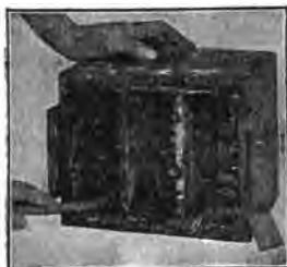
FIG. 6,319.— Battery repairs 19. Invert the case over a sink and thoroughly clean the cells by inserting a hose and injecting a stream of water upward into each cell. Be sure that all sediment and foreign matter is removed from the cells before installing the plates.
