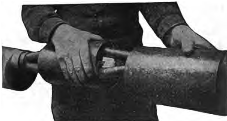
FIG. 7,414.— Cable splicing with Conducell: IV. Cell assembly held in place by the porcelain spacers and ready for the outer tube to be drawn over.
