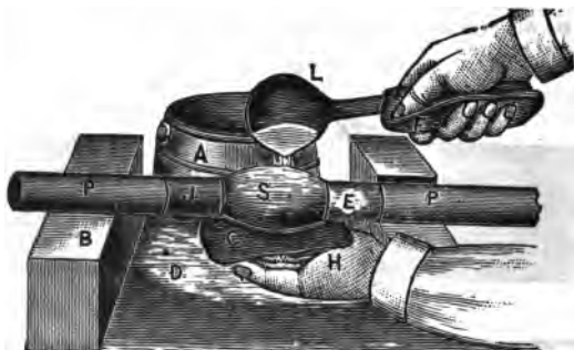
FIG. 8,605. —Method of wiping a horizontal joint. The cloth used for wiping is a pad of mole-skin or fustian about four inches square made from a piece twelve inches by nine, folded six times, and sewed to keep it from opening; the side next the pipe is saturated with hot tallow when used. If the lead has been brought to the heat of the solder, and the latter properly manipulated and shaped while in a semi-fluid or plastic condition, the joint gradually assumes the finished egg shaped appearance. In making the joint a quantity of solder is taken from the pot by means of the ladle, the solder being previously heated so hot that the hand can be kept within two inches of its surface. The solder is poured lightly on the joint, the ladle being moved backwards and forwards, so that too much solder is not put in one place. The solder is also poured an inch or two on the soiling, to make the pipe of proper temperature. Naturally the further the heat is run or taken along the pipe, the better the chance of making the joint. The operator keeps pouring and with the left hand holds the cloth to catch the solder, and also to cause the same to tin the lower side of the pipe, and to keep the solder from dropping down. By the process of steady pouring the solder now becomes nice and soft and begins to feel shaped, firm and bulky. When in this shape and in a semi-fluid condition the ladle is put down, and, with the left hand, the operation of wiping, as illustrated, is begun working from the soiling towards the top of the bulb. If the lead cool rapidly, it is reheated to a plastic condition by a torch, or a heated iron. When the joint is completed, it is cooled with a water spray, so that the lead shall not have time to alter its shape.
