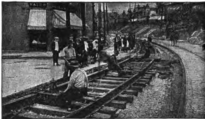
FIG. 7,925.—Chicago "Little Giant" electric track-drills reaming joint holes on the tracks of the Pittsburgh Railways Co.
